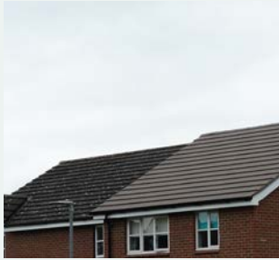
Gable roofs with varying shades of grey slate tiles
