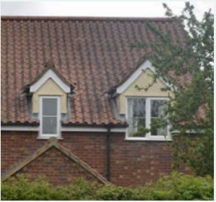
Gable dormer windows of varying sizes inset with white uPVC framed windows
