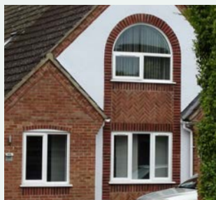
Brick detailing around fenestration including a soldier course curved lintel
