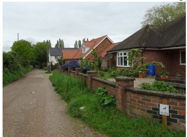
Figure 29: Development that offers a good variety of vernacular style, mass and roof type.
