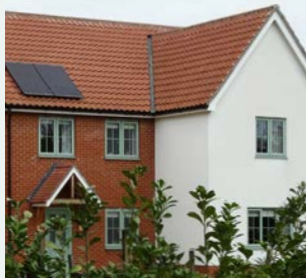
Single dwellings utilising a variety of facade materiality such as brick and render
