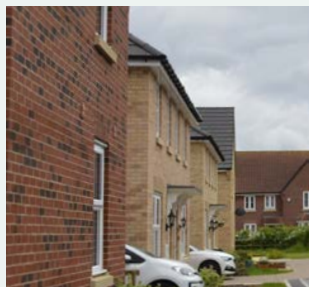
Variety of brick colouring including red, brown and sand with darker accent bricks
