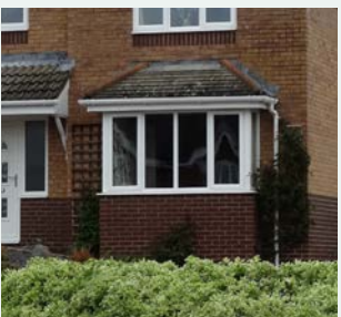
Square bay window with dual casement panels and a hipped roof
