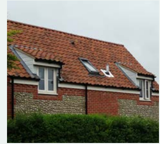
Two evenly spaced shed roof dormer windows with double casement frames
