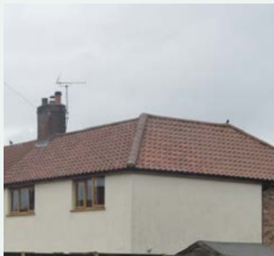
Hipped roof with consistent height across neighbouring dwellings
