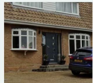
Bow windows of varying sizes and diamond muntin pattern on upper panes
