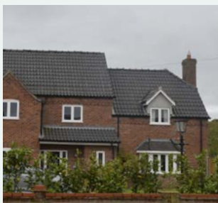
Mix of roof types and heights including additions such as a dormer window
