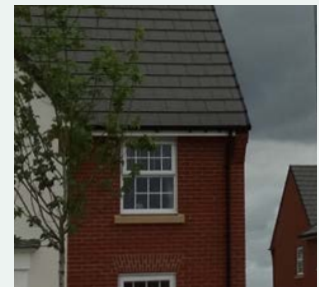
White uPVC mock sash window with a grid pattern mullion and brick lintel
