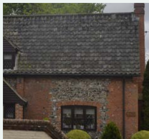
One of a few examples of a facade featuring rubble flint between red brick
