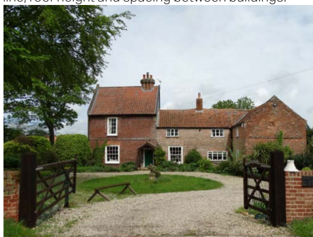
Figure 23: The Lindens is a good example of sensitive rural character such as in its setback, boundary treatment and permeable paving.
