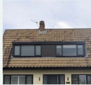
Long flat roof dormer casement window with dark grey framing throughout facade
